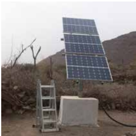
Photo: Example of solar panels used to power well pumps in Djibouti; Shade garden example. UNDP
