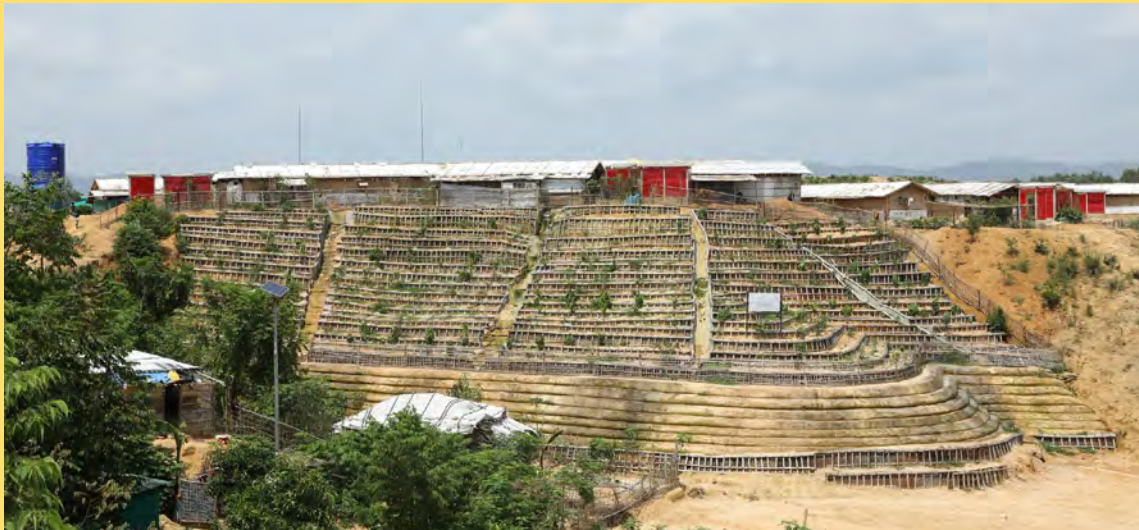
Bangladesh - Land stabilization is essential to protect Rohingya refugees from landslides during the monsoon season. ISCG/ Syed Md Tafhim
